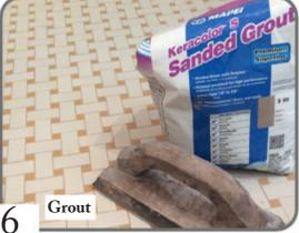
Use sanded grout, keep grout float flat with tile surface, do not overwipe and create shallow joints. Wait 72 hours for curing. Reseal all tile/grout as needed. For more information: refer to the TCNA Manual (Tile Council of North America), current edition for tile installation standards and methods.
