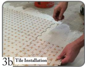
Lay one sheet at a time. Check alignment and consistency of spacing between sheets.
