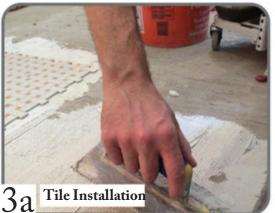
Apply mortar using a 1/8"- 3/16" V-notch or U-notch trowel for tiles 2"or smaller. Work 2-4 square foot section at a time to prevent mortar skim over.
