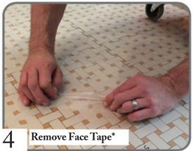
Wait a minimum of 12 hours before removing face tape. Pull plastic off at the horizontal (against tile). A heat gun can be used 6-8 inches from floor to loosen bond.
