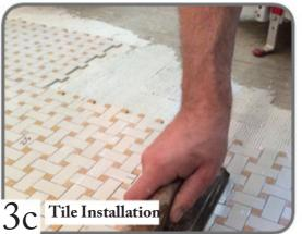
Use a grout float, speed square or block of wood to push tiles flat into mortar while setting. Repeat step 3 until all sheets are laid. Let dry.
