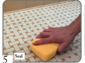
Use water to remove any hazing or residue. Seal all porcelain tile and allow to dry a minimum of 12 hours.
