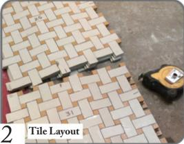
Dry laying the tile is recommended. Adjust the pattern and cut the tiles to fit the space. Number the sheets and stack them for quick and correct installation.
